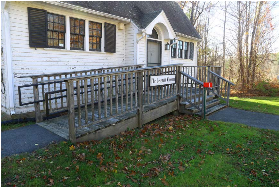
Fig. 20. North elevation showing the access ramp and steps.
