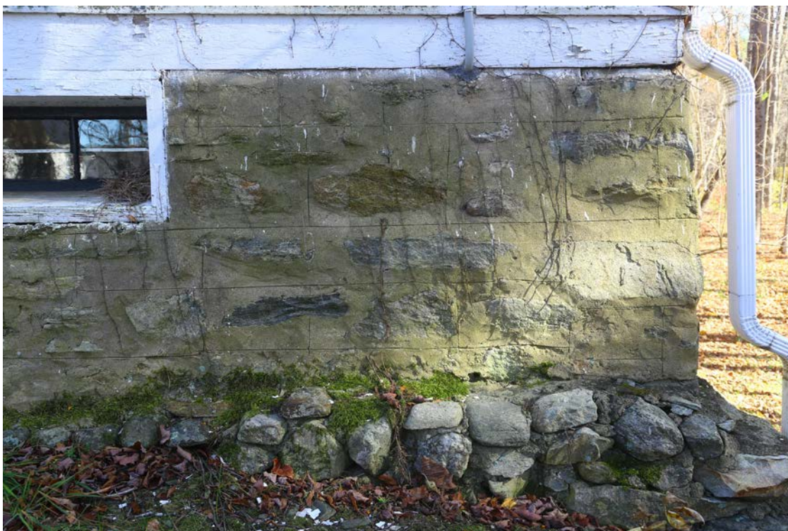
Fig. 19. Typical treatment of the foundation. The foundation shows areas of exposed rubble stone, with rendered masonry above in some locations. The render is struck to create the appearance of joints, giving the impression that the foundation is constructed of coursed stone.
