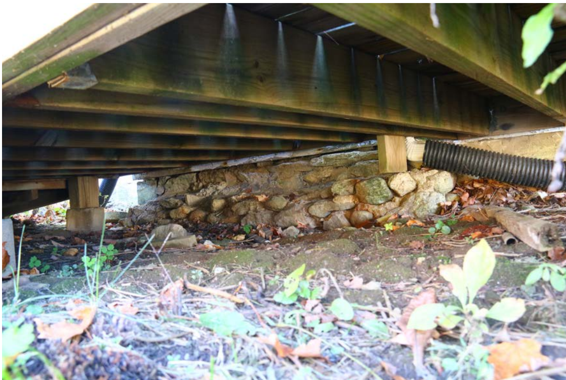
Fig. 25. View under the north deck showing the remains of the original steps into the building.
