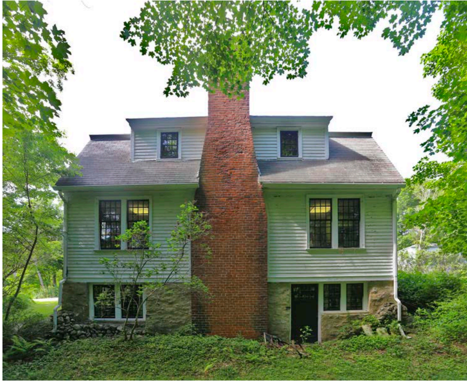
Fig. 3. South elevation. July 2025.
