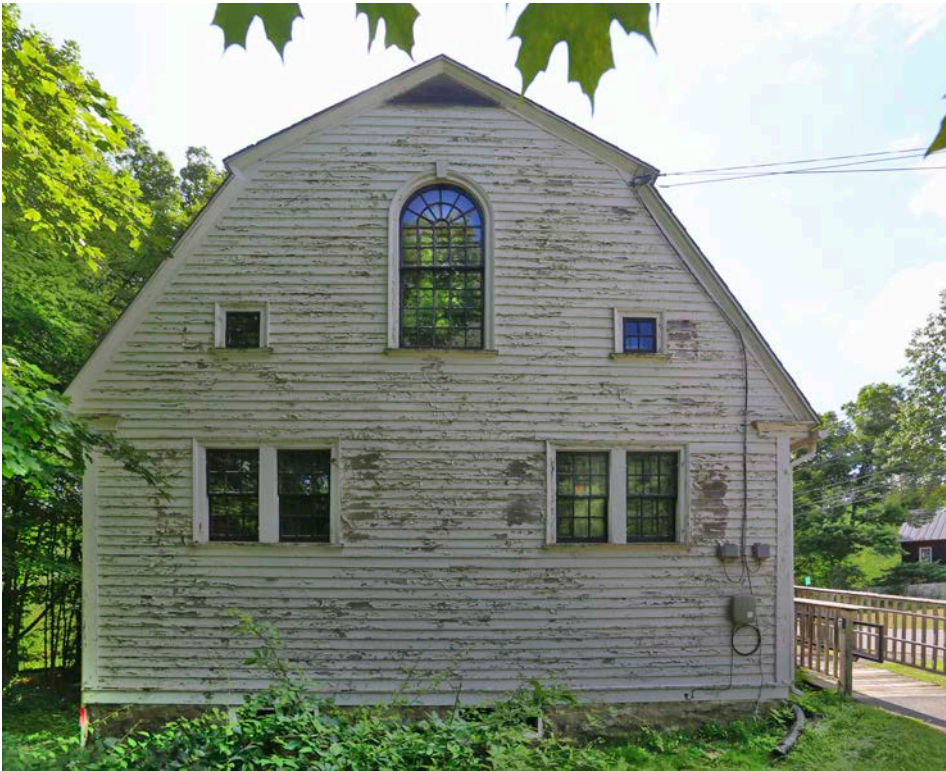
Fig. 4. East elevation. July 2025.
