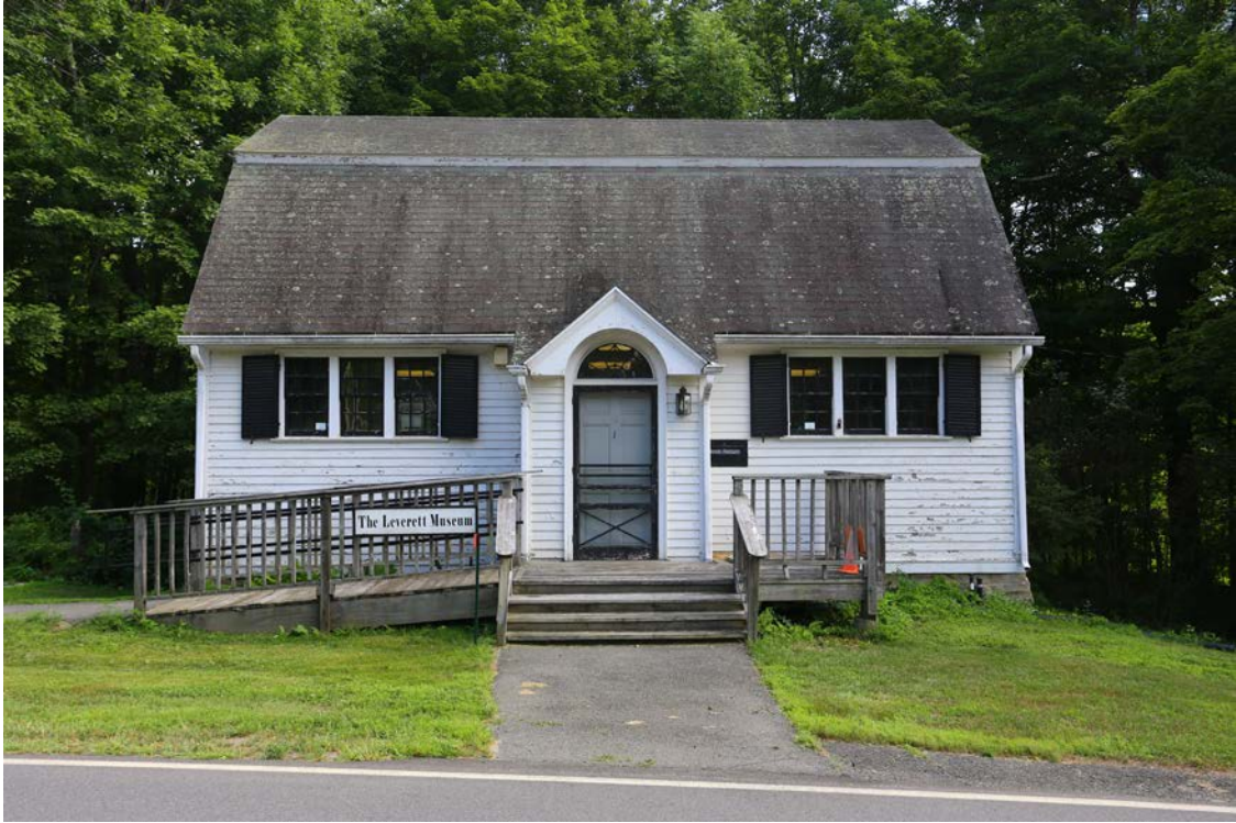
Fig. 1. North elevation. July 2025.
