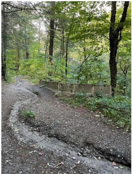
The stone wall foundation of the road has fallen into the ravine in three places. Two barriers have been put at the edge of the road and a third location fenced.
