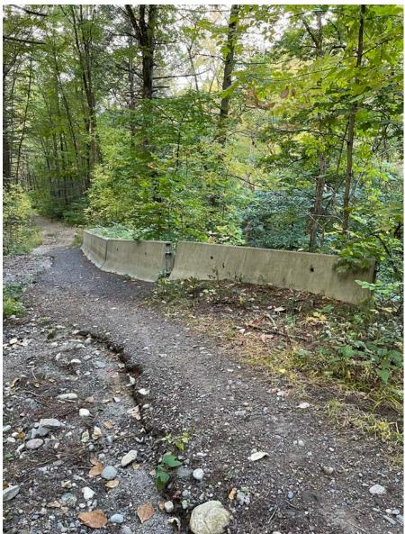
Rattlesnake Gutter Road was built circa 1834. Using oxen to move rocks, they built a stone wall and then backfilled it with dirt to make the road. During the "100 year flood" of 1993, a small section of the road was undercut and the stone wall breached. It has grown larger over the years and the town has put up three barriers at the edge.
