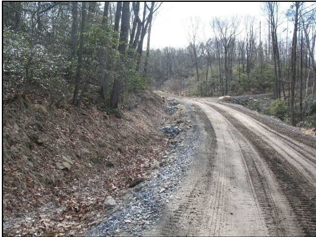
Stone check dams at construction site.
