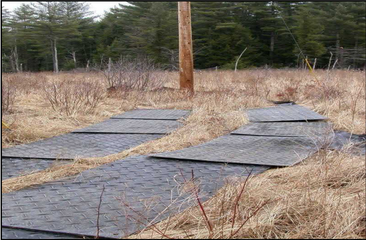
AlturnaMAT® tracks to utility pole in wetland.
