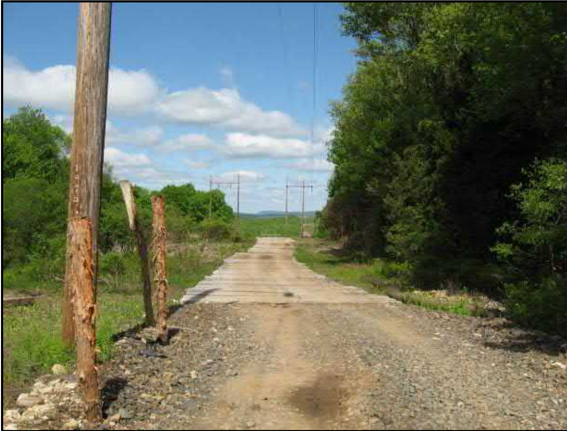
Construction mat access road.
