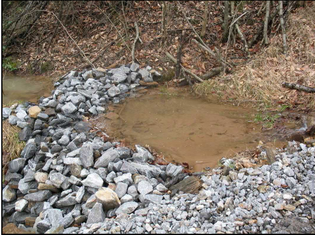
Stone check dam at construction site.
