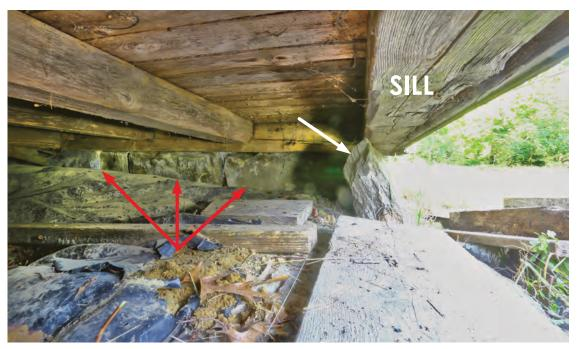
Fig. 16. South elevation at east end of the building where stone in Figure 14 is missing. View looking east. Tilted stone (white arrow) is the same seen in Figure 14. Red arrows point to foundation stones on the east side of the building.
