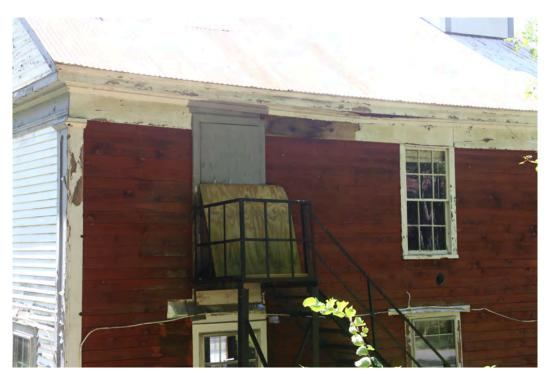
Fig. 10. North elevation showing area of rotted soffit. The corner and portions of the surrounding trim and siding here should be opened up to expose the full extend of conditions shown in Figure 5.
