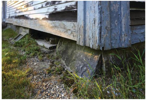
Fig. 14. Detail of the foundation at the southeast corner of the building. Note missing stone and tilted angle of the corner stones.
