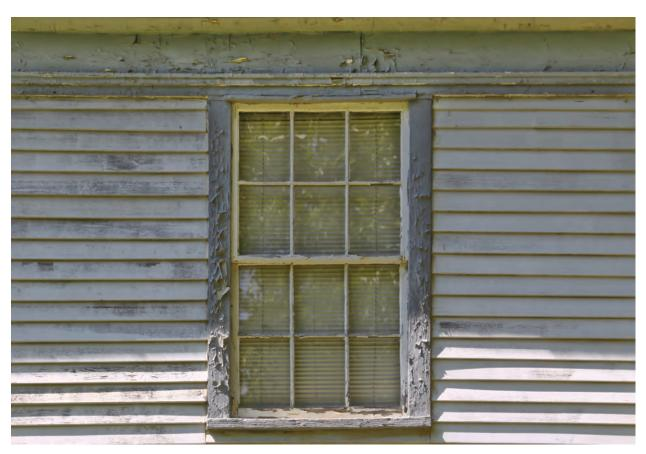
Fig. 12. Representative example of the typical exterior conditions of the wood frame windows. Note the failing paint finishes and missing glazing putty on the sash.
