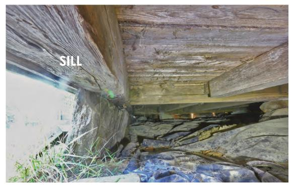
Fig. 15. South elevation at east end of the building where stone in Figure 14 is missing. View looking west. Note how sill bears on foundation stone.
