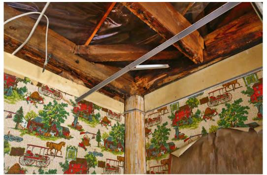
Fig. 5. Second floor, northeast corner. Detail of rot at the top of the corner post and ends of wall plates.
