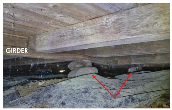
Fig. 17. Detail of the girder supported by piles of stone.
