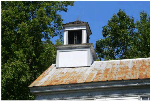
Fig. 6. Detail of the bell tower and surrounding metal roofing. Rusted surface of the roofing is typical across the entire roof.
