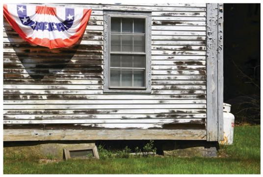
Fig. 7. South elevation, east corner. Representative appearance and condition of clapboard siding and wood trim elements.
