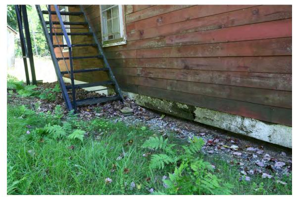
Fig. 18. North elevation. Note how high the grade is in relation to the water table. The grade should be slightly lowered and pitched away from the building. This section of water table (approximately 16') should be replaced.
