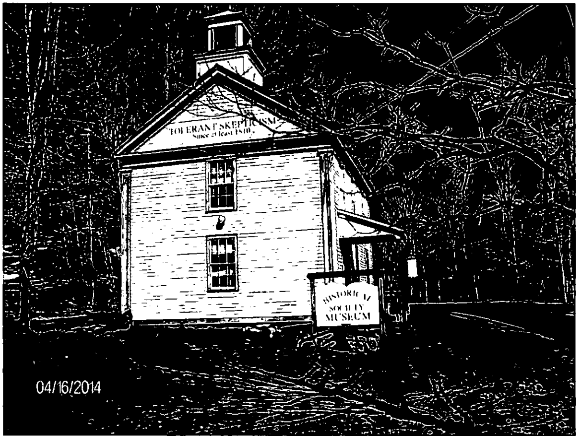
1. West and south elevations of Schoolhouse (Apr. 16, 2014)
