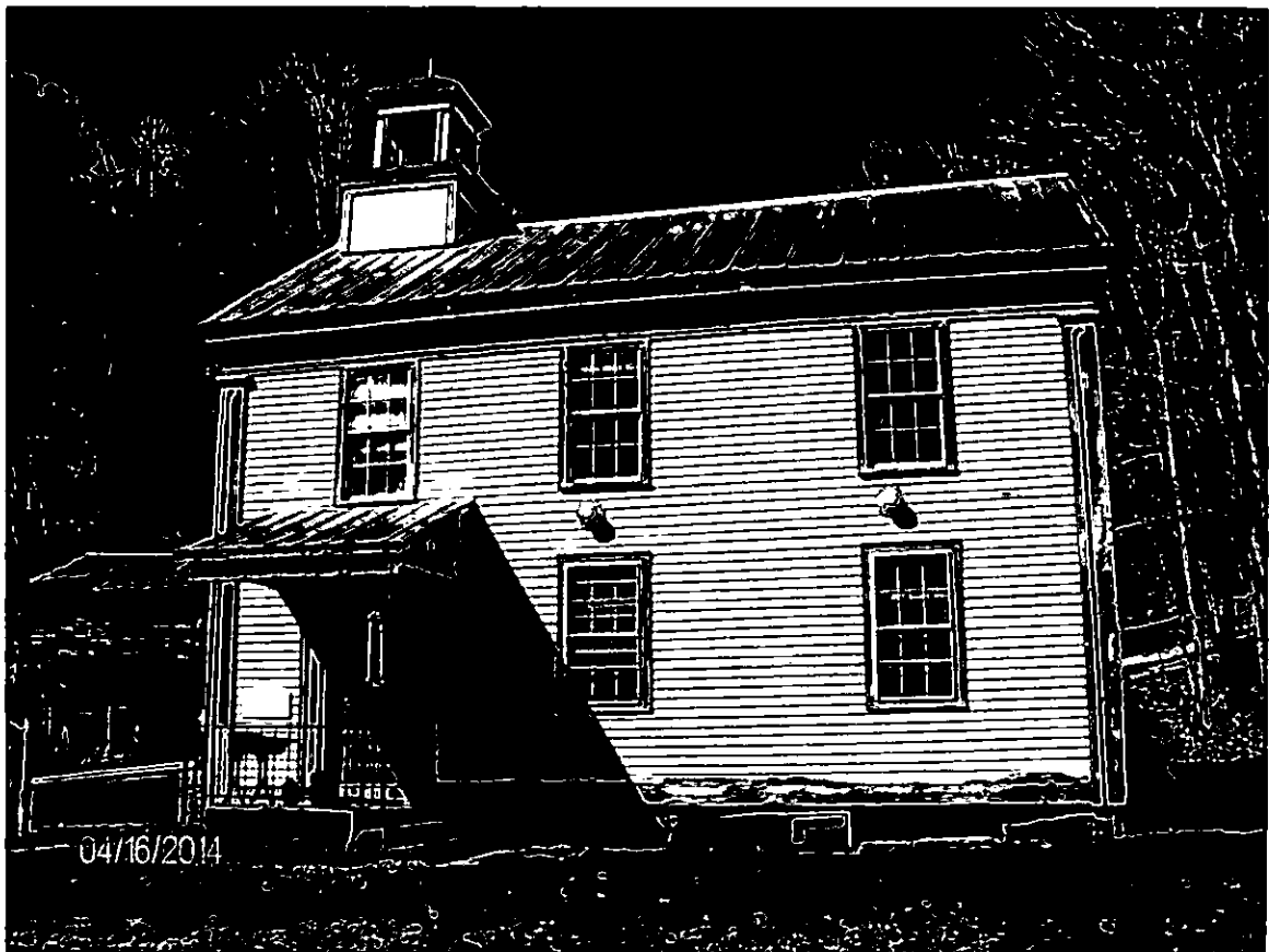
2. South elevation of Schoolhouse (Apr. 16, 2014)
