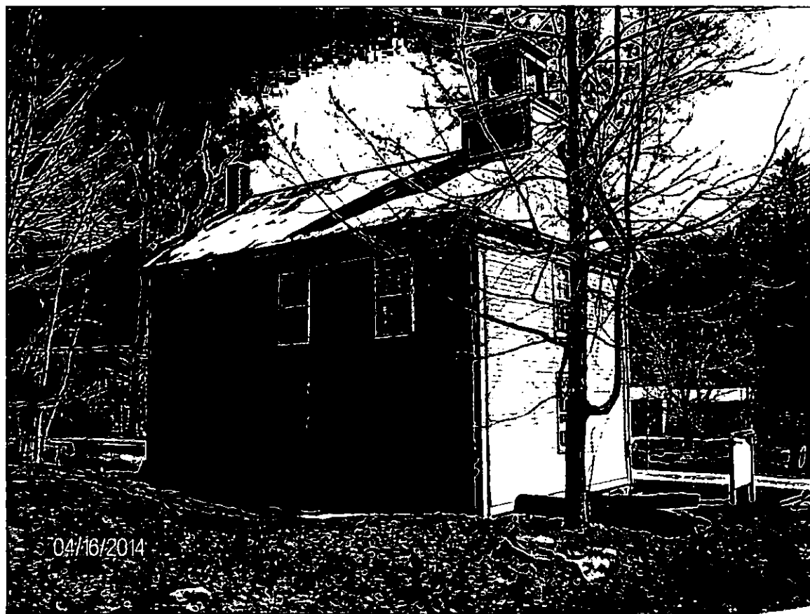
6. North and west elevation of Schoolhouse (Apr. 16, 2014)
