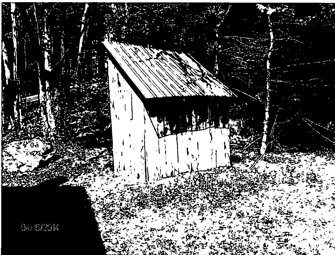
4. West and south elevation of Outhouse (Apr. 16, 2014)
