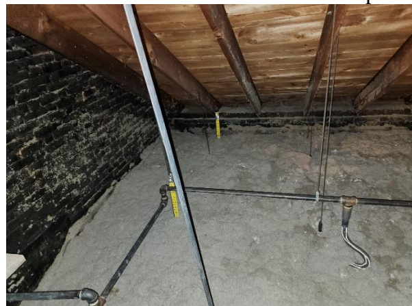
Older Attic AIP Insulation Depth
