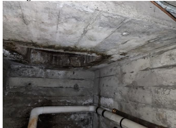
Green Door Crawlspace - thin fiberglass on ceiling, uninsulated water pipes present.
