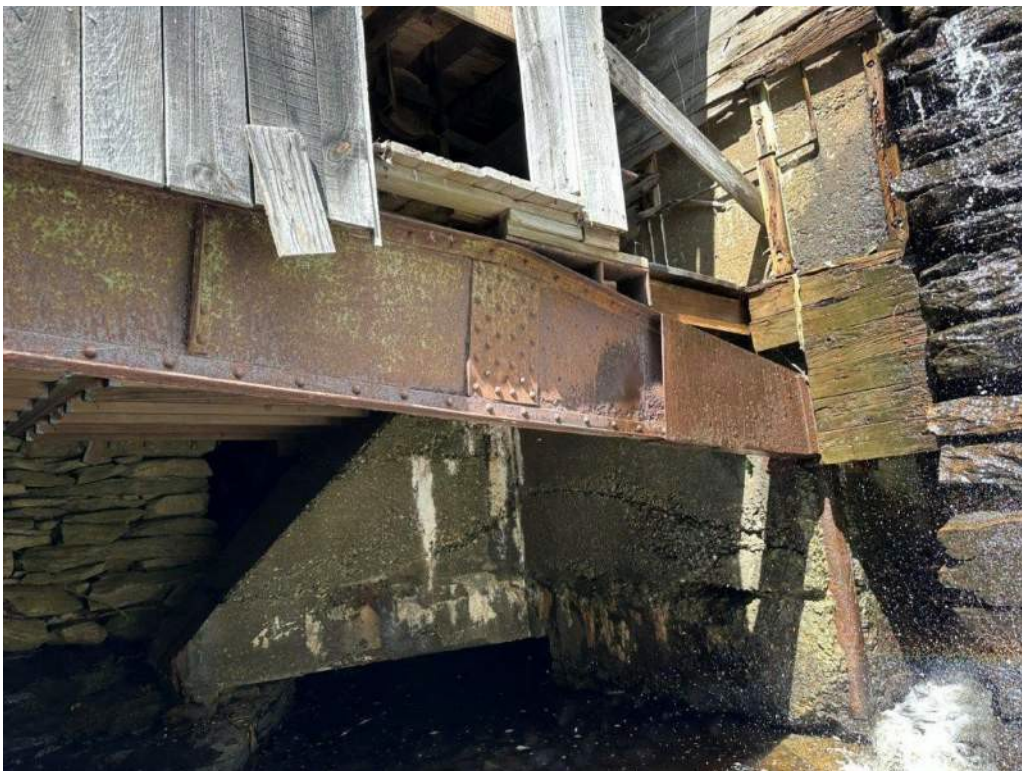
Photo 2 Rusting beam at south elevation with poor continuous floor support
