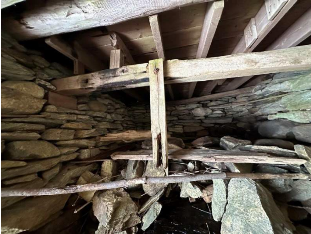
Photo 1 Poorly supported and rotted joist ends
