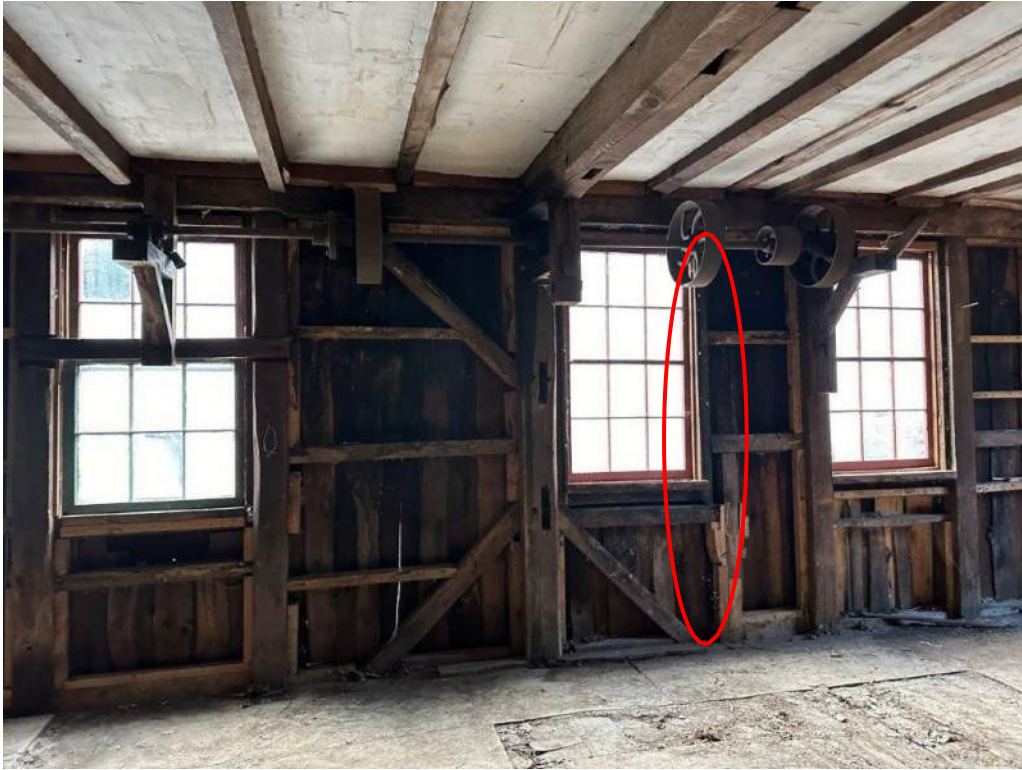
Photo 3 Missing window stud
