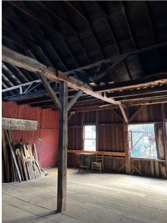
Photo 5 Spliced timber beam
