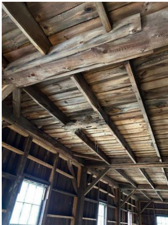
Photo 6 Scant framing at loft level
