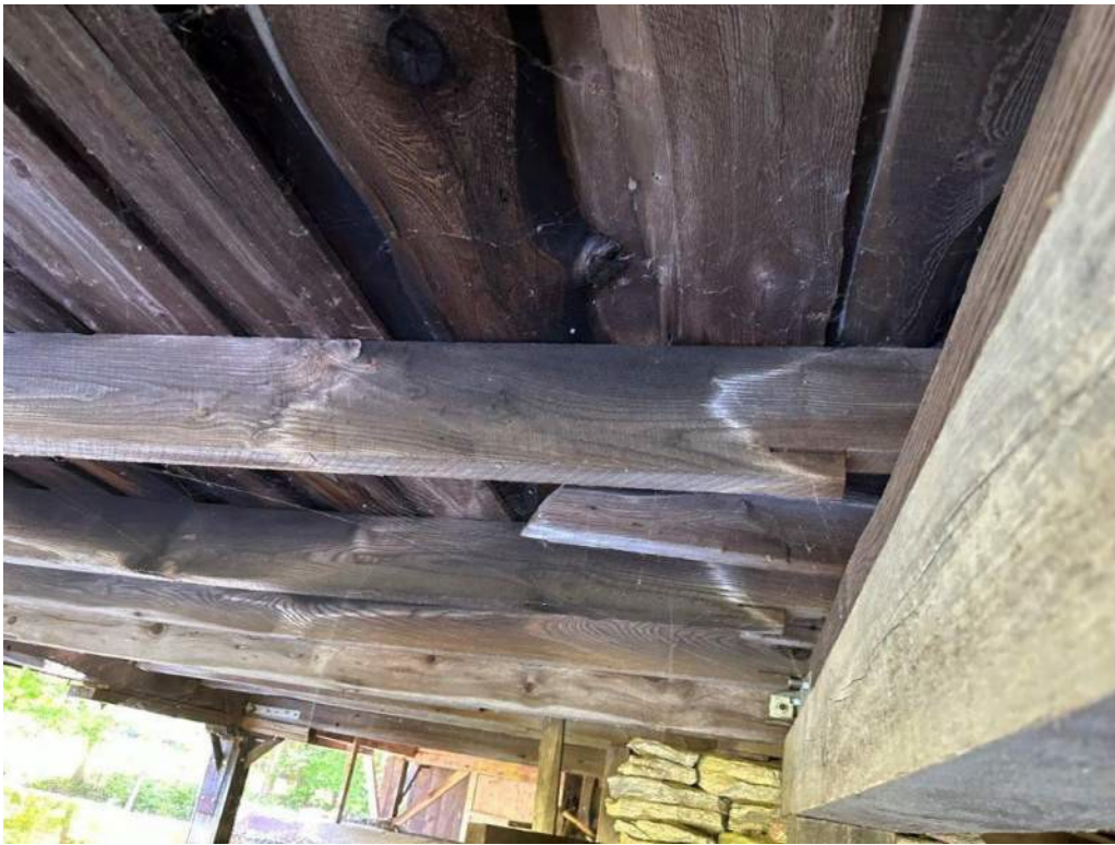
Photo 4 Notched floor joist
