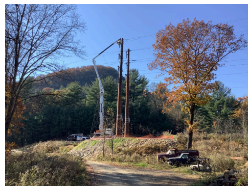
Photo No. 6 STR 10089 line work in progress, facing west.
