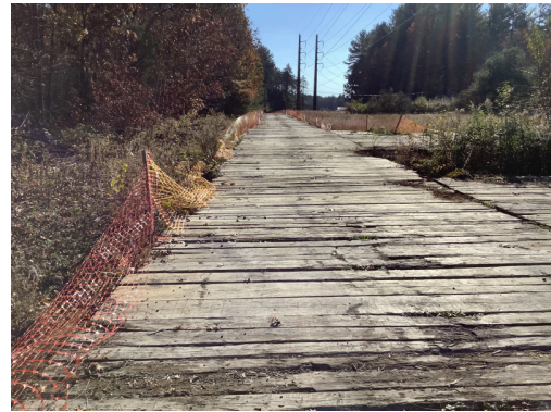
Photo No. 2 STR 10084 repairs to cultural fencing are needed, facing south.
