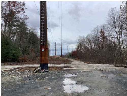
Photo No. 15 STR 10133 facing south.
