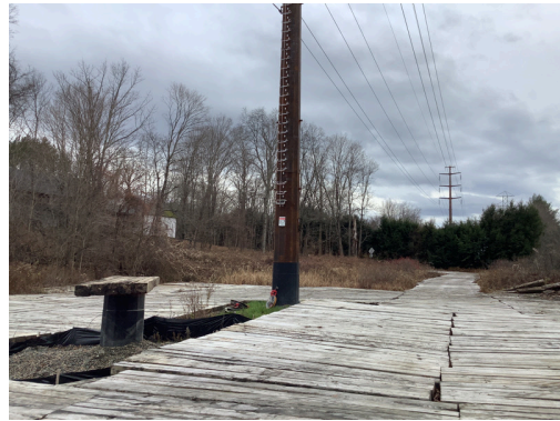
Photo No. 14 STR 10128 facing south.
