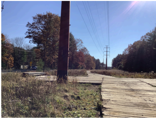
Photo No. 1 STR 10083 line pull complete, facing south.
