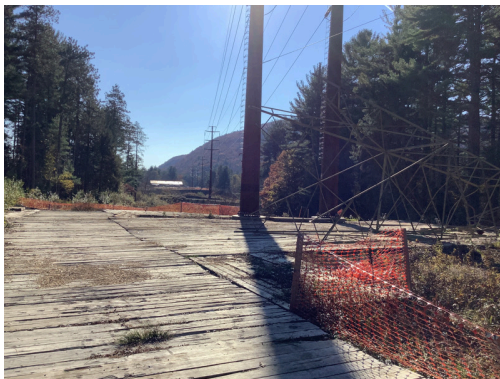
Photo No. 3 STR 10085 line work complete, facing south.
