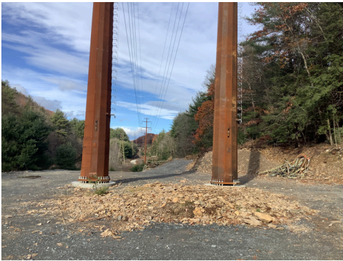
Photo No. 7 STR 10100 facing north, line work complete.
