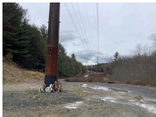
Photo No. 12 STR 10122 line work complete, facing north.
