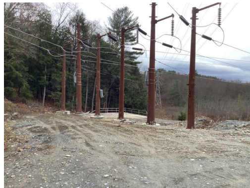
Photo No. 10 STR 10119 line work complete, facing east.
