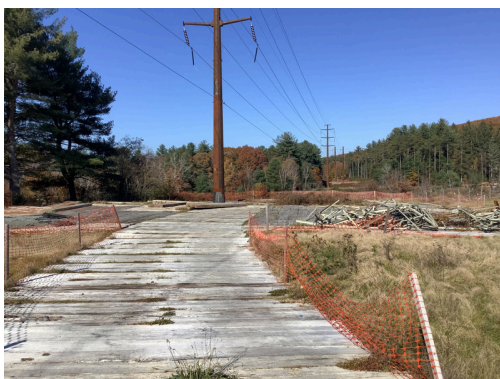
Photo No. 5 STR 10087 line work complete, facing north. Repairs to cultural fence are needed.
