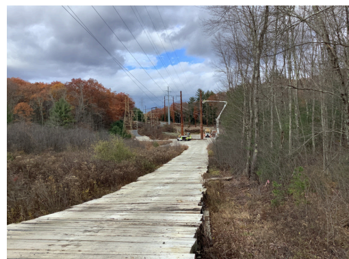
Photo No. 12 STR 10119 - 10137, line work in progress.
