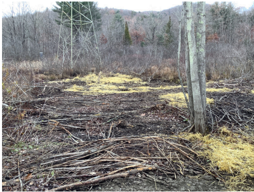
Photo No. 7 STR 10109 civil restoration in progress, facing west.
