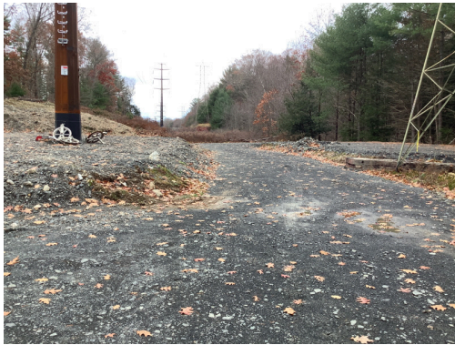
Photo No. 13 STR 10124 line work complete, facing south.
