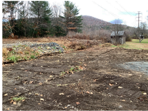
Photo No. 8 STR 10111 civil restoration in progress, facing north.
