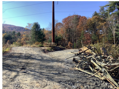
Photo No. 4 STR 10086 line work complete, facing west.
