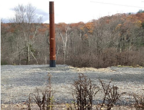
Photo No. 9 STR 10108 facing east.
