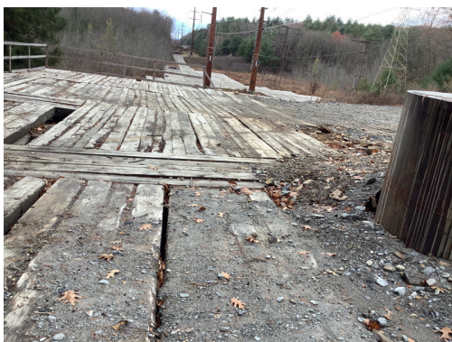
Photo No. 11 STR 10119 sweep mats and refresh erosion controls near stream.
