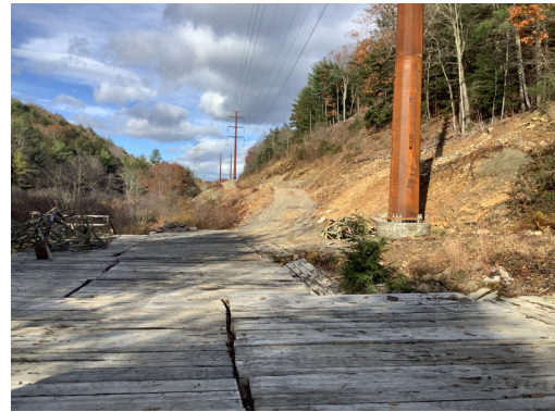
Photo No. 8 STR 10102 facing north. Line work complete.
